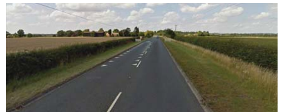
1.2. View of A4129 Thame Rd.
