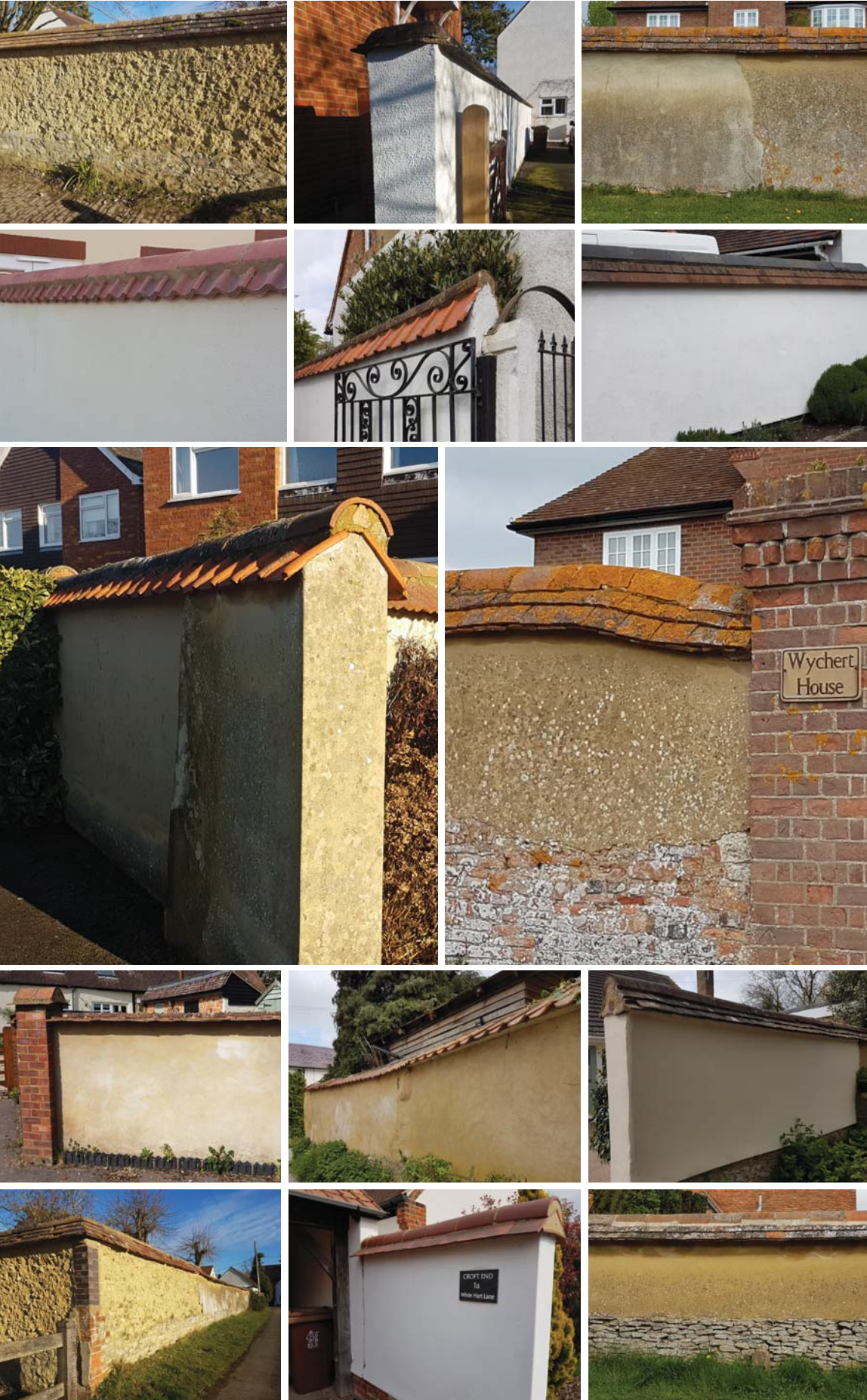
5.3. Variation of existing Wychert Walls across Haddenham
