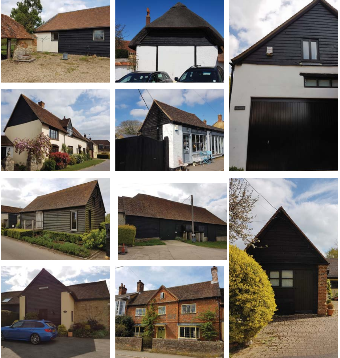
5.4. Photographs of local town show fully boarded buildings, combinations of black weatherboarding with white/cream render and local brick
